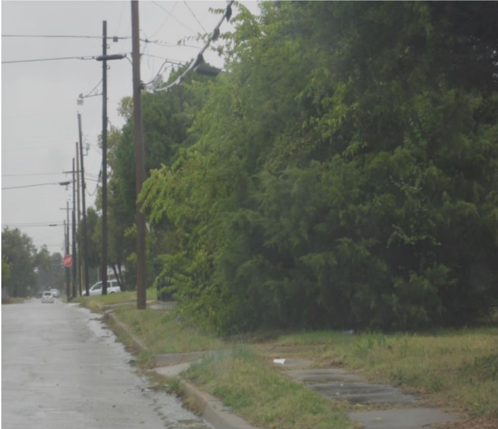
Figure 2.40: Overgrowth over sidewalks
