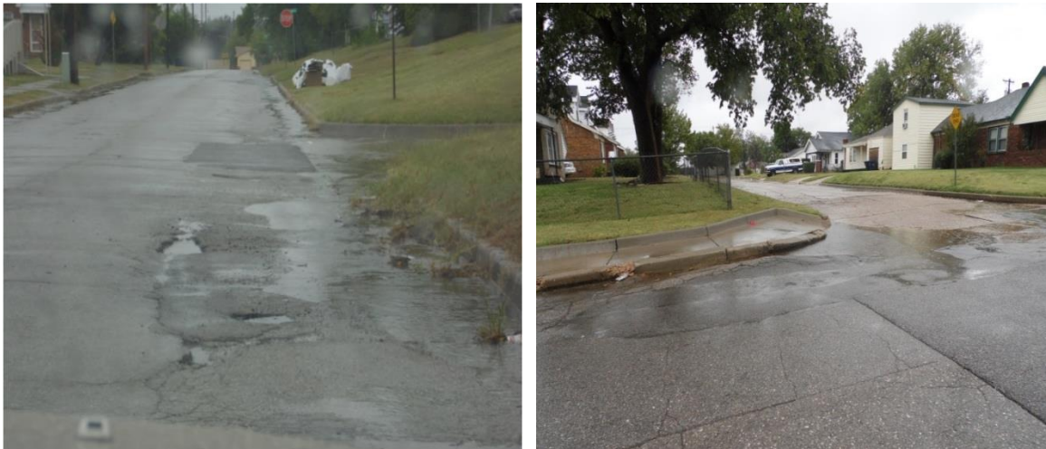
Figure 2.41: Road Condition Examples
