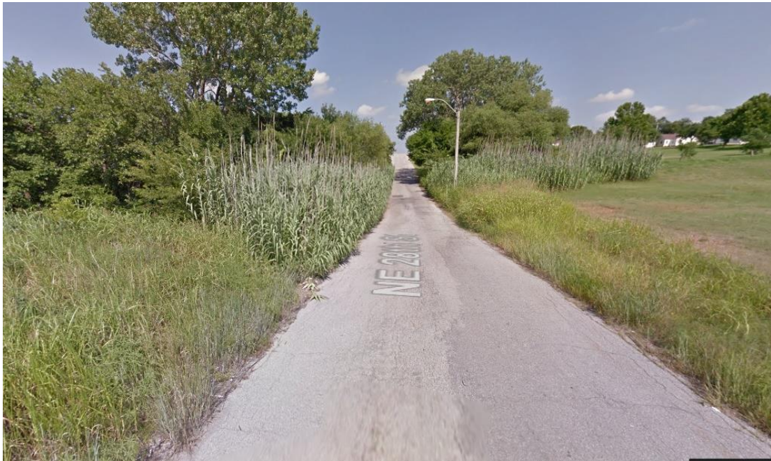
Figure 2.31: View of NE 28 th West of Harden Park (Google)
